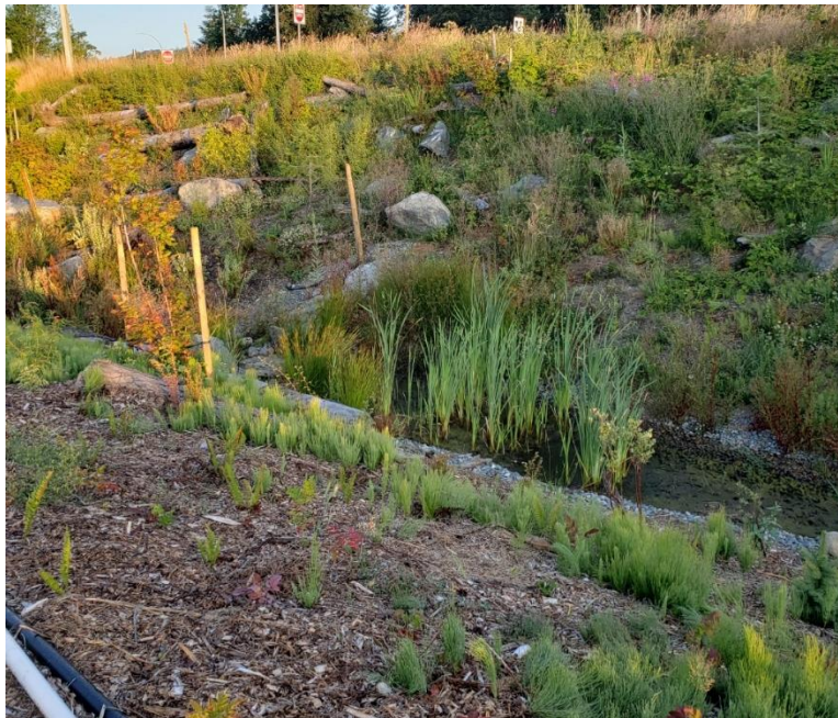
Stream restoration along Burnside Road (Ann Nightingale)
