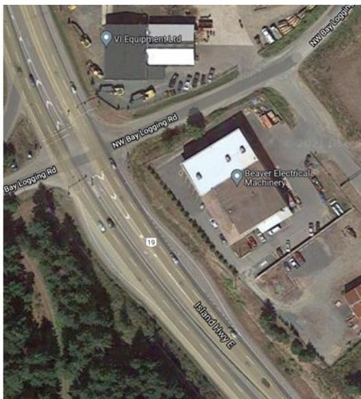
Island Highway and NW Logging Road
