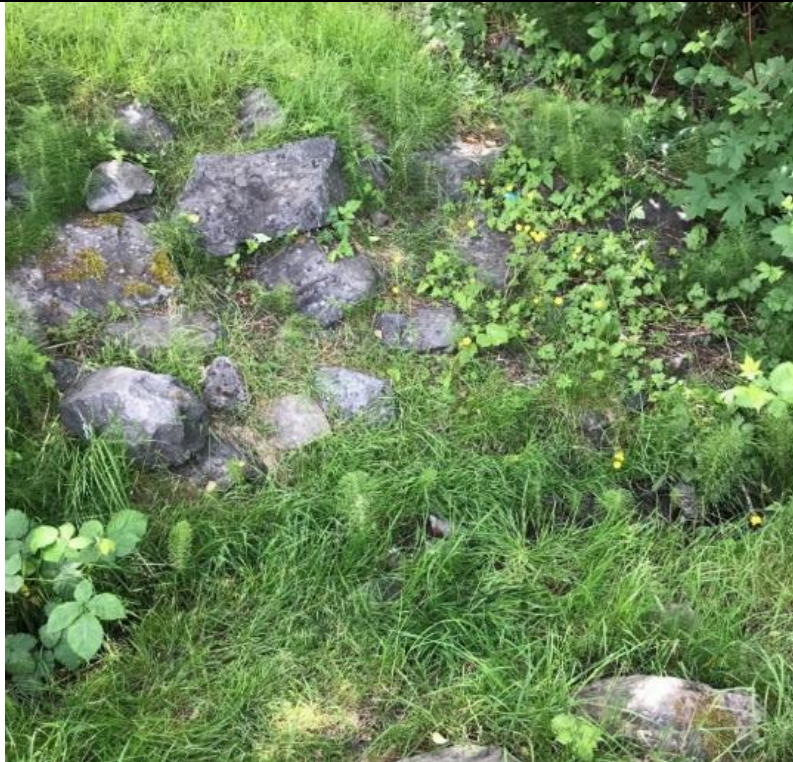
Photo 14 Watercourse 3 south of Watkiss Way showing rock armouring on banks.
