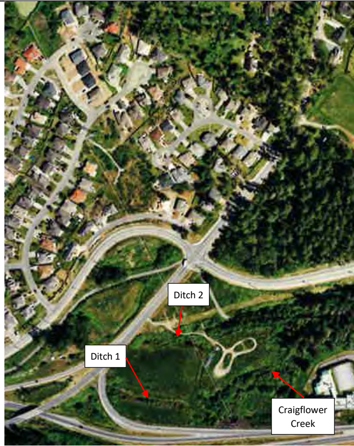
Air Photo – 2005: Site conditions after the construction of the Burnside Road offramp from Highway 1.
