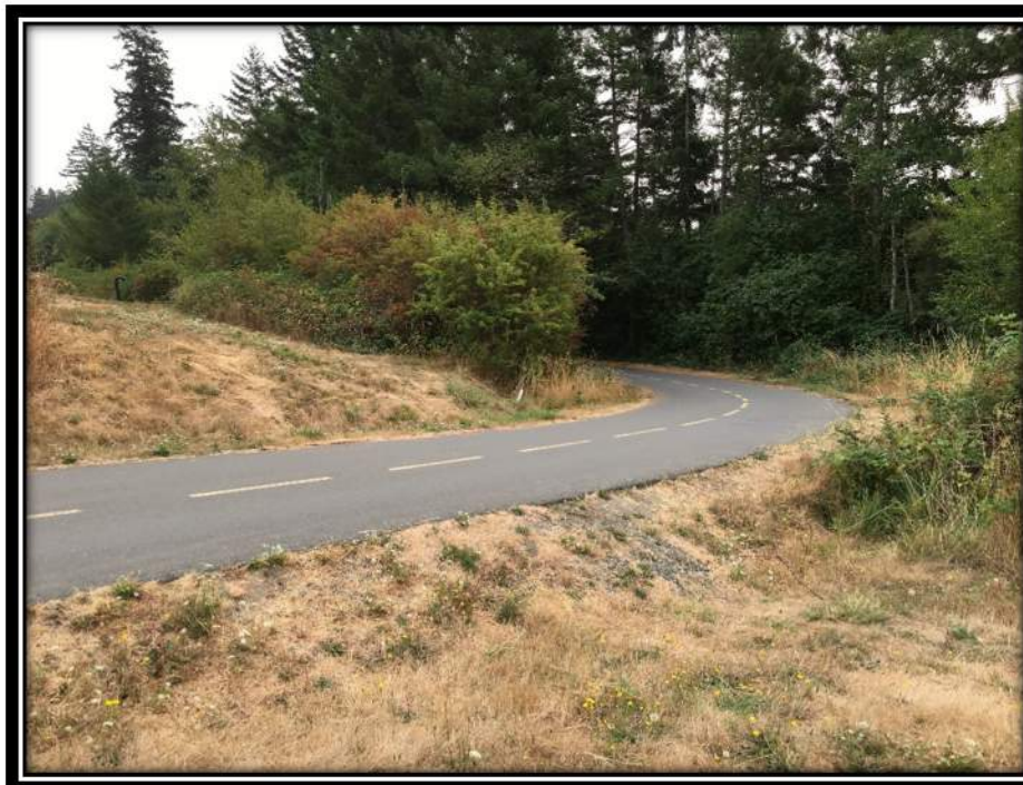
Photograph 6: Photo showing a portion of the former Canadian National Railway, currently the Galloping Goose Trail (APEC #5). Photo looking east.
