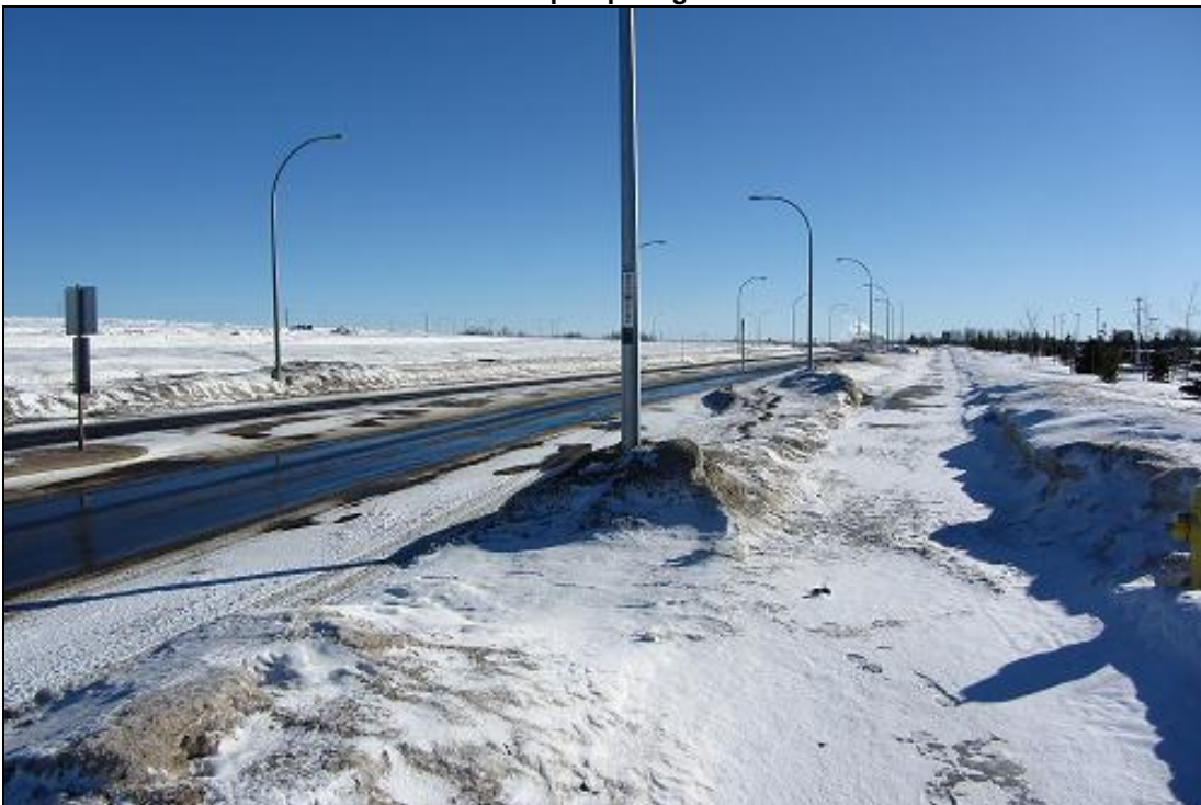
Photo 3: Bus stop requiring snow removal
