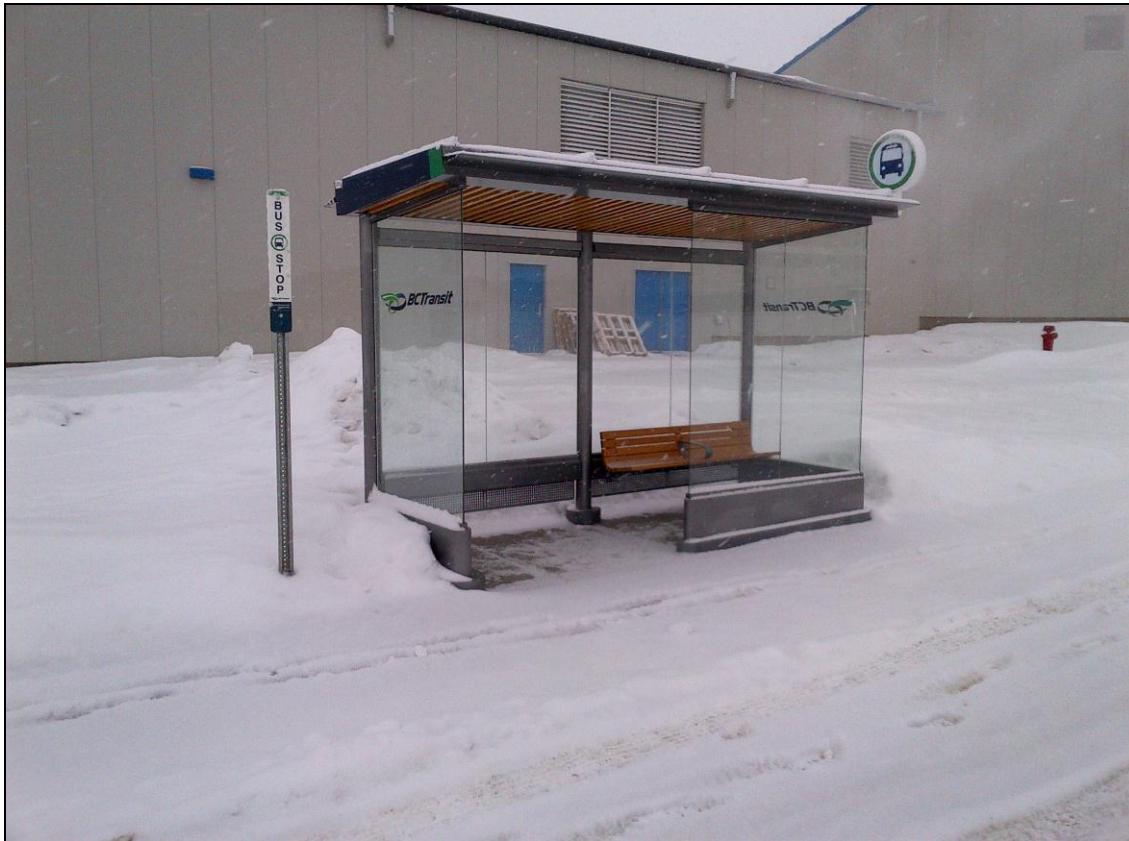
Photo 4: An example of a new bus shelter
