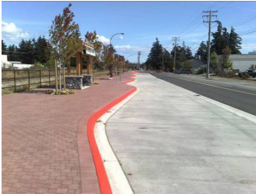
Figure 5.4 Sawtooth Loading Platform
