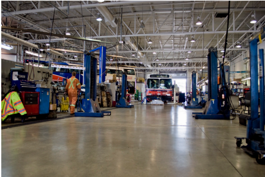
Langford Transit Centre Facility
