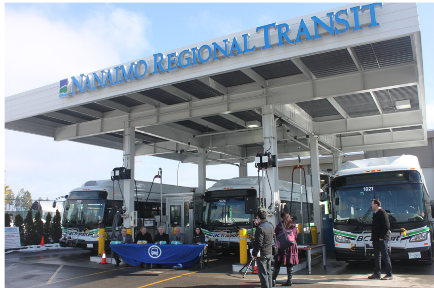
CNG Fueling station with CNG buses in Nanaimo
