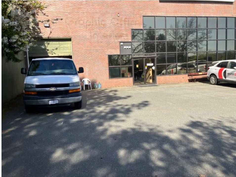
Photograph No.1: View of the front of the office building
