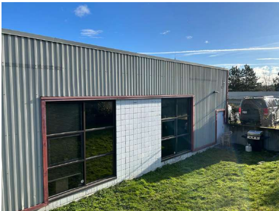
Photograph No.1: View of the exterior of 4210 Commerce Circle
